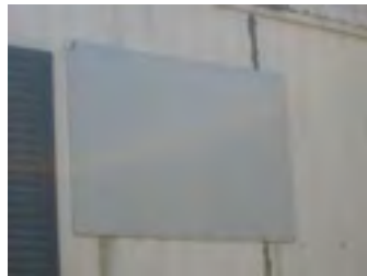
Sheet metal panels by Joe Ervin
